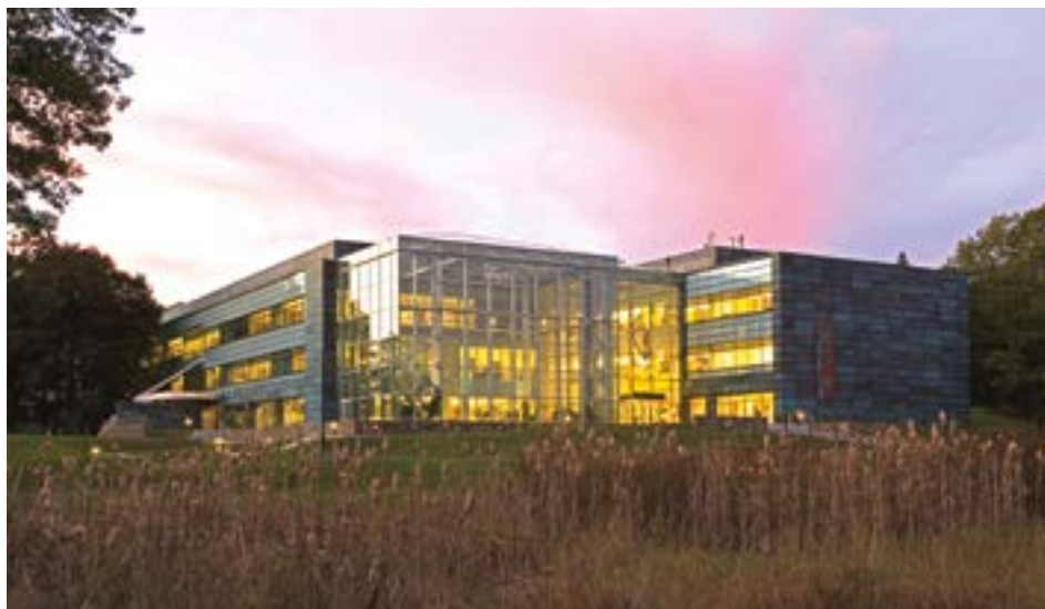
NEB Headquarters in Ipswich, MA, is LEED-certified and designed with sustainability in mind.
